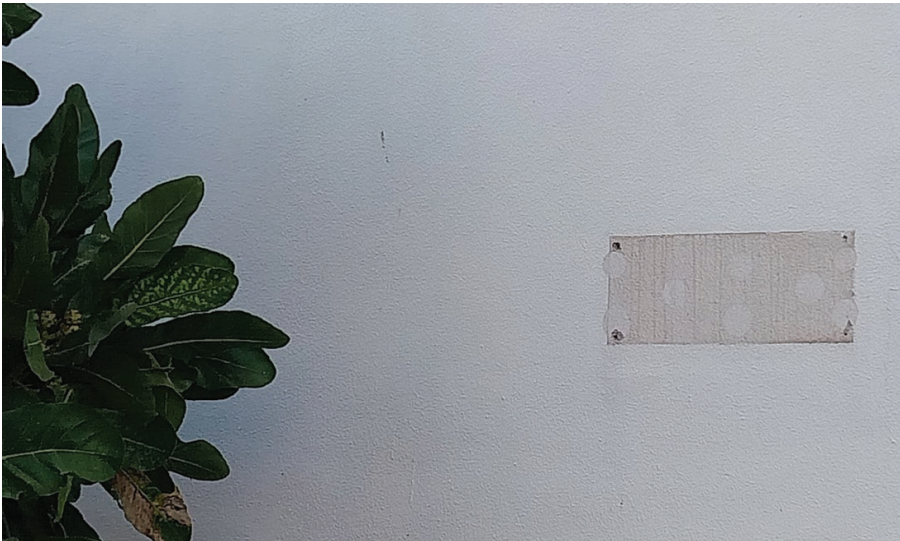
Figure 3.3. Calle Alejandro Cioranescu missing sign on the gentrified hotel building (personal photo, August 2023)
