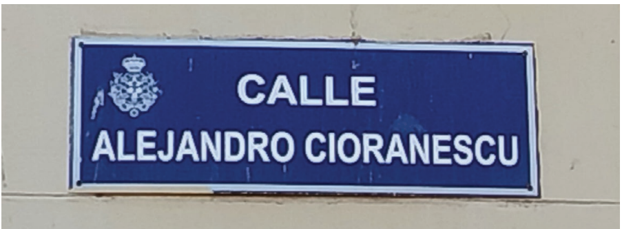
Figure 3.2. Calle Alejandro Cioranescu sign on the delapidated Edificio José Fumero (personal photo, August 2023)
