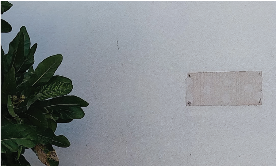
Figure 3.3. Calle Alejandro Cioranescu missing sign on the gentrified hotel building (personal photo, August 2023)
