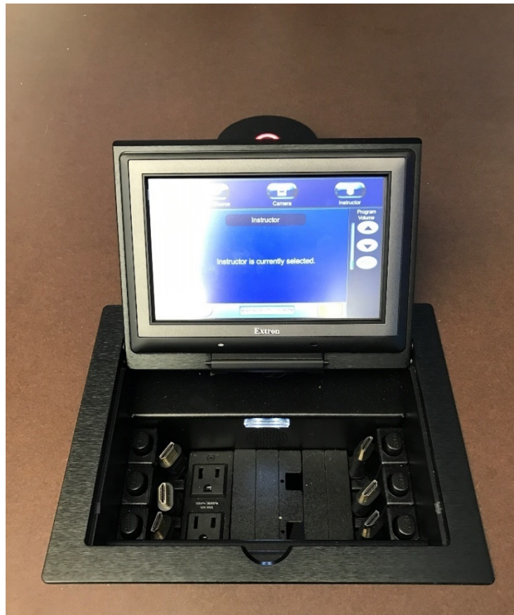
Figure 2: The control panel at each student table includes two outlets, six cable cords to connect laptops, volume control, and the ability to select from the following screens: connected laptops 1-6, the instructor’s desktop computer, and the camera mounted at each table (McClain, 2016b).
